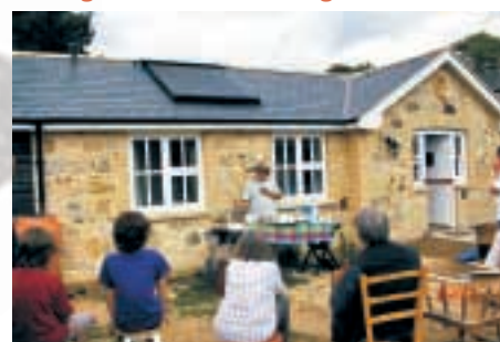
At the official opening of Studio Cottage on the Isle of Wight.
