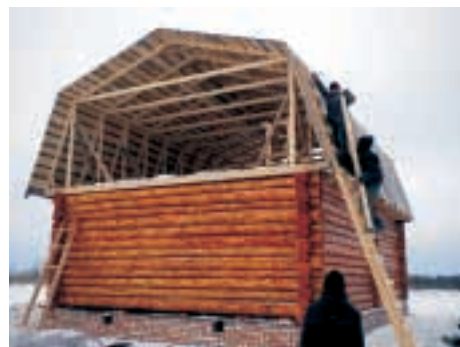
Roofing the community's first house continued despite the winter snow.
